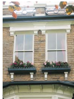
(i) Sliding sash windows constructed in timber.
